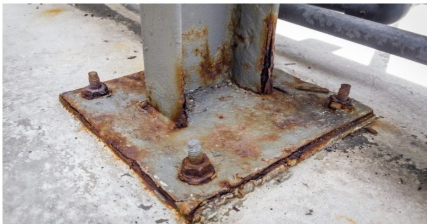
Figure 72 Crevice corrosion
