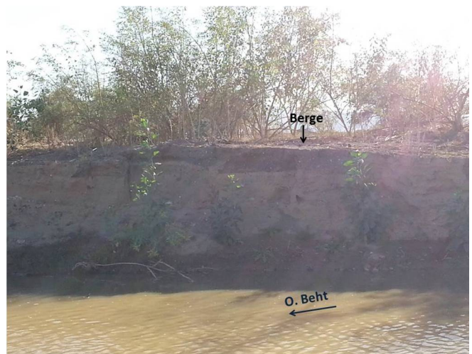
d-Berge verticale rive droite, aval autoroute A2 (6/11/2017)
