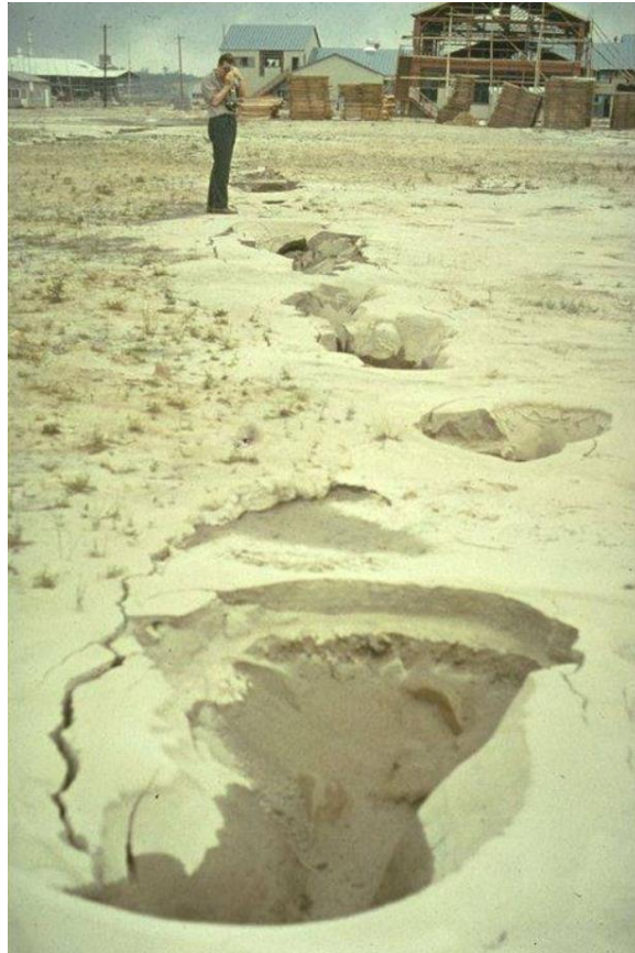
Figure 3-1: Liquefaction caused damage illustration after Niigata, japan 1964 earthquake, (a)- Building overflow, (b)- Showa bridge failure, (c)-soil liquefaction evidence on sand.
