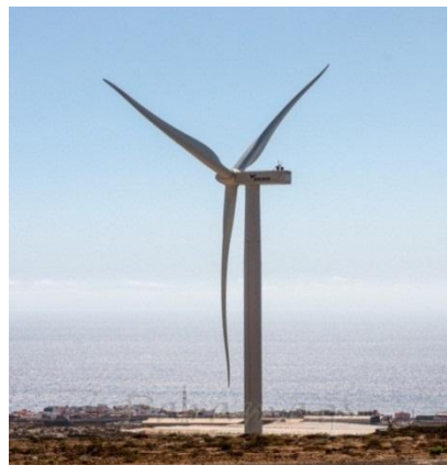
Figure 1. 4 Recent generation of wind turbines design installed (Simens Gamesa 3.47 MW, rotor diameter 132 m) [14]
