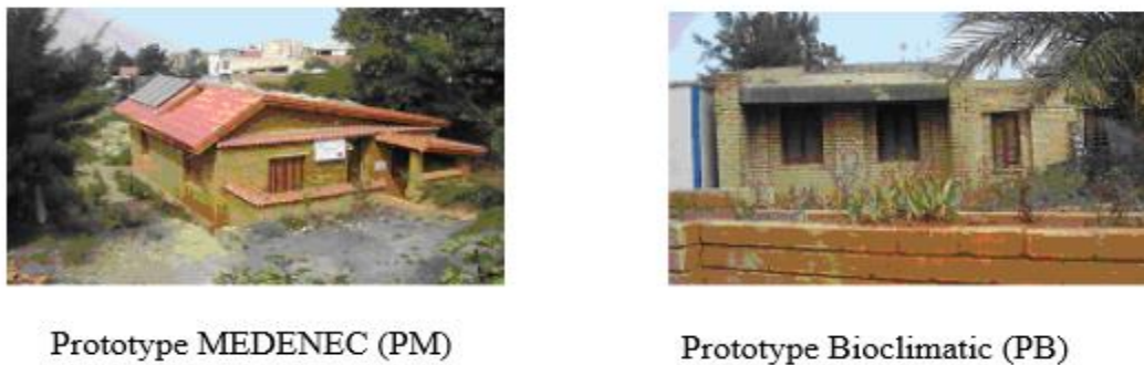
FIGURE 18. CEB BUILDINGS MADE AT CNERIB.
