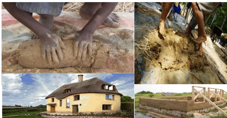
FIGURE 6. COB EARTH BUILDING TECHNIQUE BY EARTH MATERIAL.
