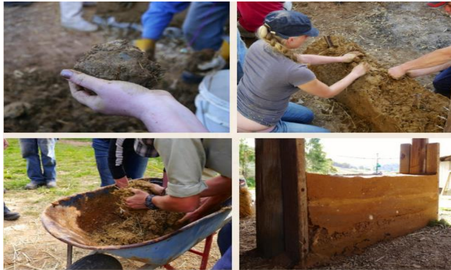
FIGURE 7. LIGHT EARTH BUILDING TECHNIQUE BY EARTH MATERIAL
