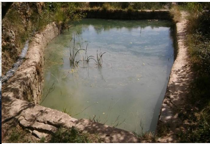
Photo 18 : Bassin de stockage (Tijent)
