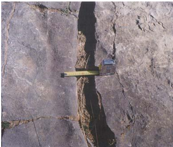
Figure 60 : Fissure de grande taille, Ibaqalliwn.
