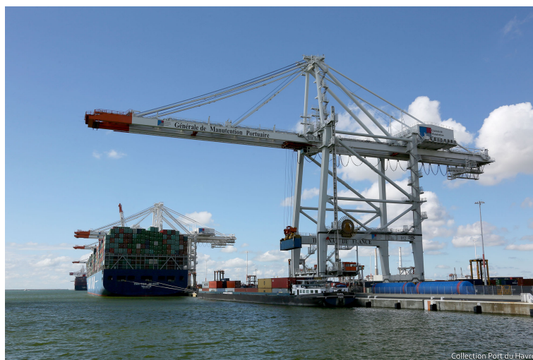
Figure I.11 – Grue de quai
