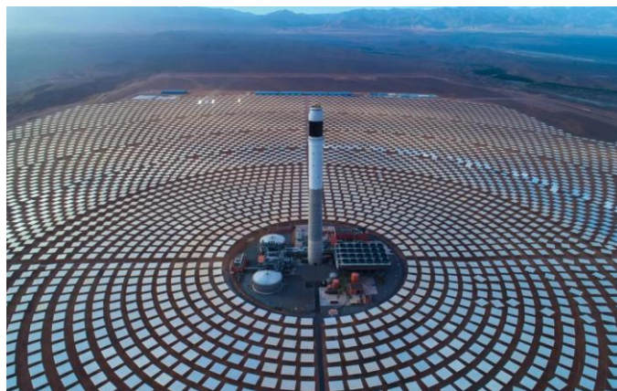
Figure 1.4 : Central solaire Noor-Ouarzazate
