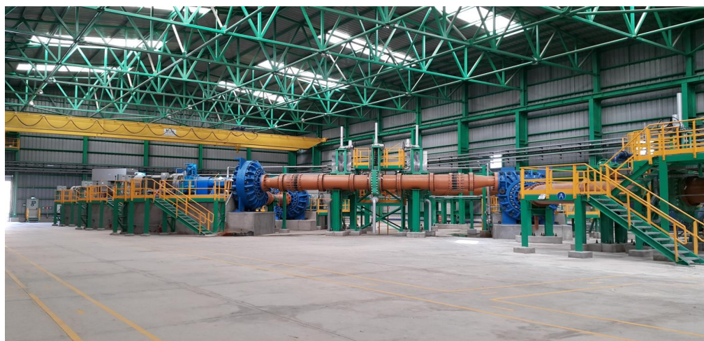
Figure 15: Centrifugal pumps in series
