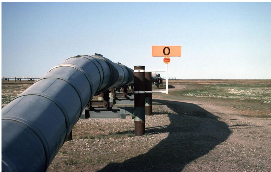
Figure 1: Pipeline linking Prudhoe Bay to Valdez, (Alaska).
