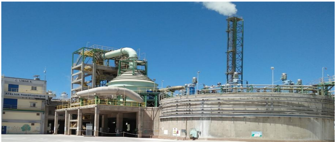
Figure 3: Photo of the attack section of line E
