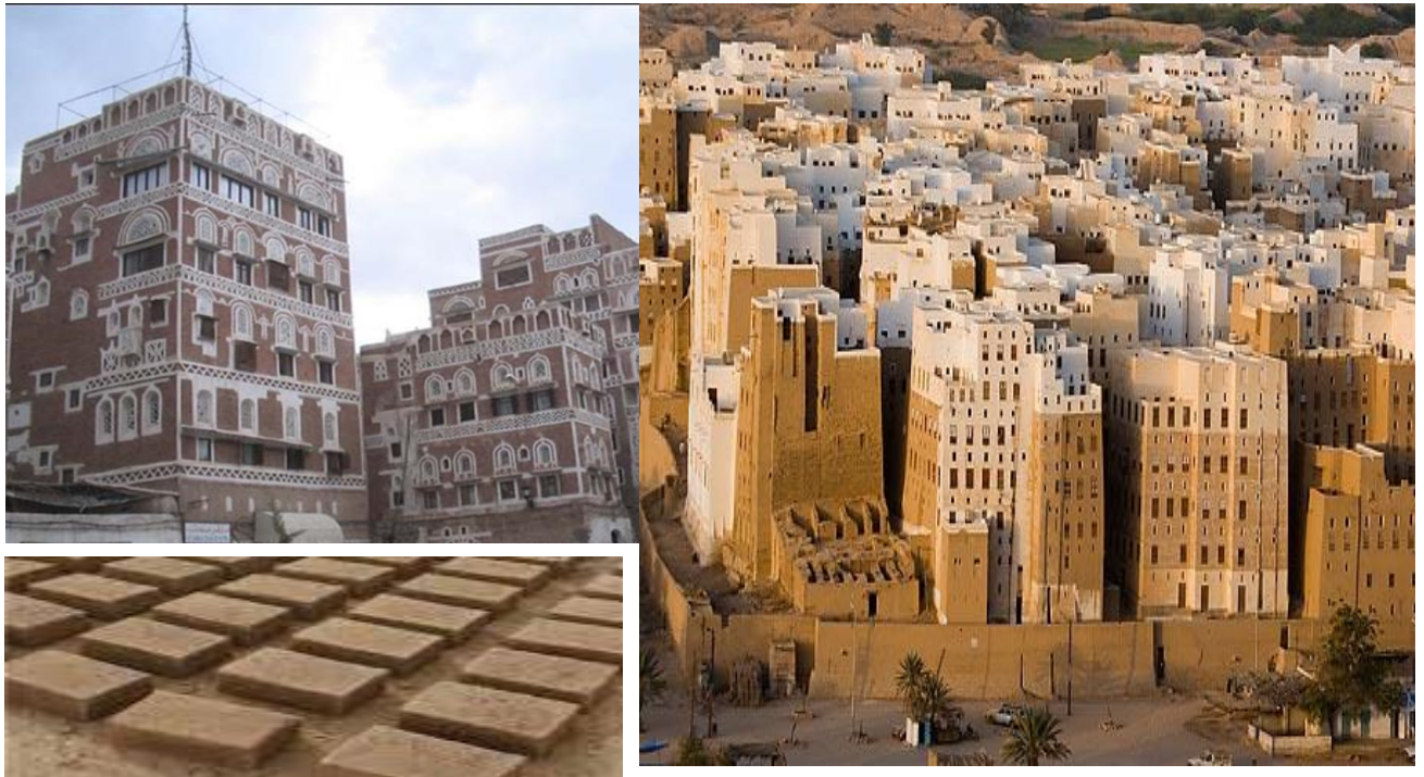
Fig. 3- 5: Homes made of mud in Yemen
