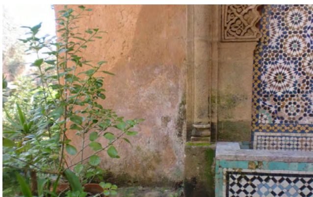
(a) efflorescence
