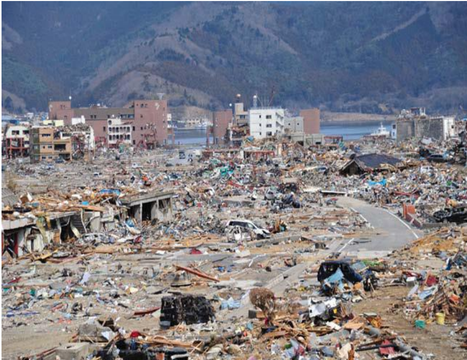
Figure 19: total collapse of constructions in Onagawa area. Near the coast, engineered reinforced concrete constructions can be seen damaged but standing. 2011 [141].
