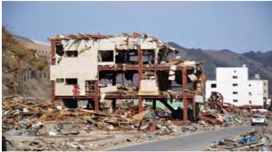
Figure 92: total deformation of steel frame building elements in Onagawa city E. Lekkas[233]
