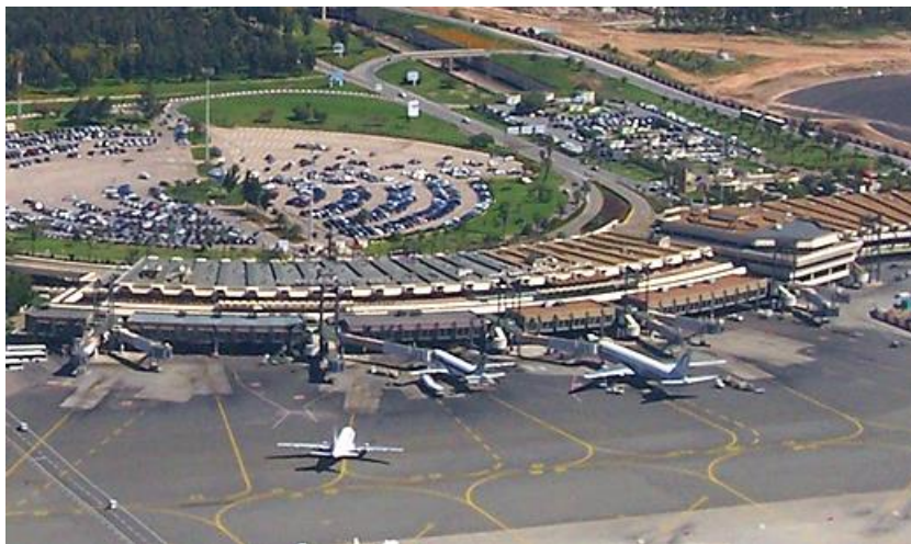
Figure 31 Example of gating at Mohamed V airport
