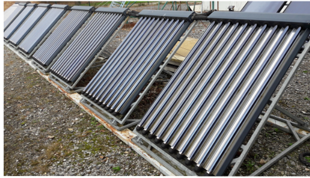
FIGURE 2.23: Solar thermal collector's field using Evacuated Tubes Collectors (ETC) technology
